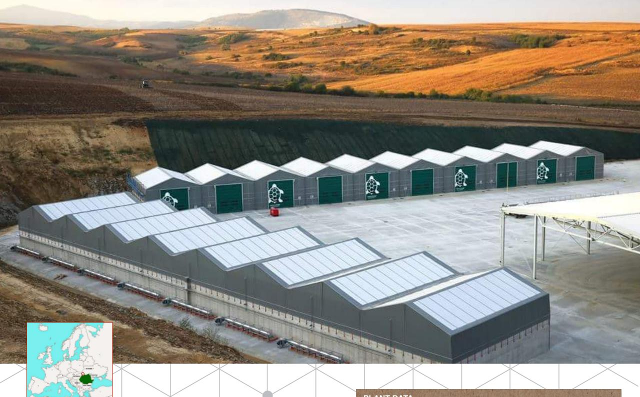
WITH THE **TURTLE™ BIOCELLS SYSTEM**, ENTSORGA ENABLED THE COMMUNITY OF GALDA DE JOS AND THE PROVINCE OF ALBA JULIA TO MANAGE MORE EFFICIENTLY **MUNICIPAL SOLID WASTE** BY PREPROCESSING MSW PRIOR TO LANDFILLING. THIS SUBSTANTIALLY **IMPROVED THE ENVIRONMENTAL IMPACT** OF THE DISPOSAL SYSTEM BY REDUCING VOLUMES LANDFILLED, LEACHATE PRODUCED AND RELEVANT GREENHOUSE GASES EMISSIONS.
